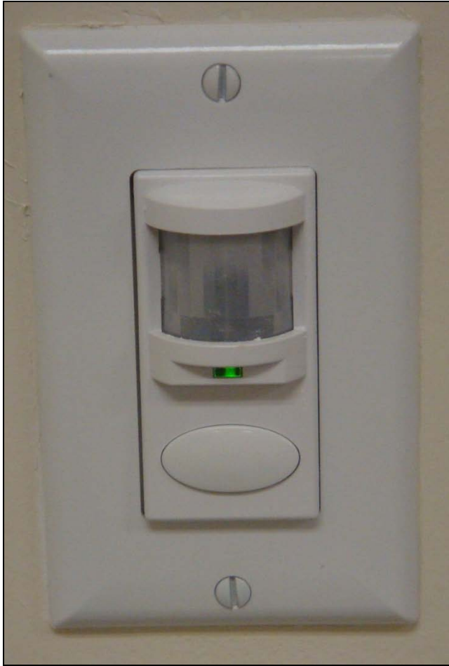
Wall Mounted Motion Sensor to control lighting
