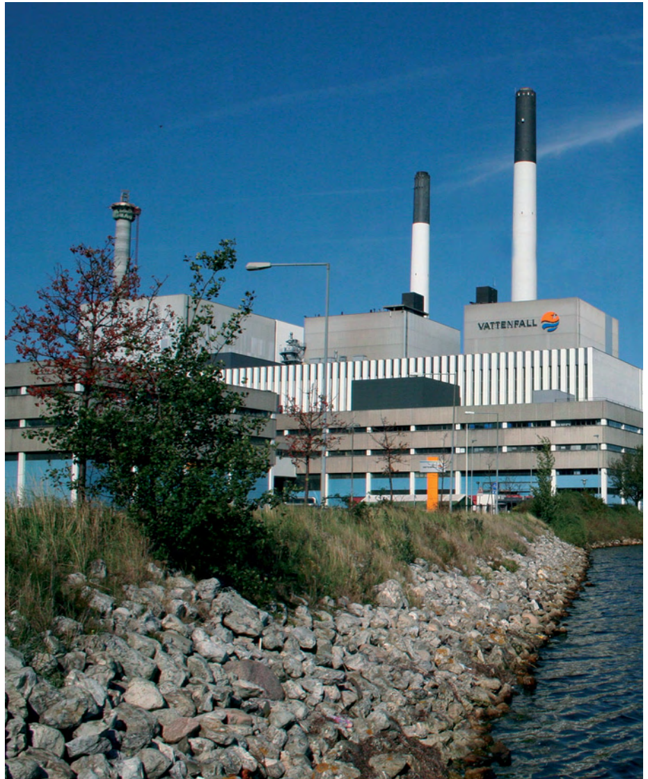
Amagerværket Power Plant (AMV), owned by Vattenfall. During 2004-9 unit 1 was thoroughly renovated and equipped to burn biomass as well as oil and coal. A geothermal demonstration plant is located at Amagerværket.
