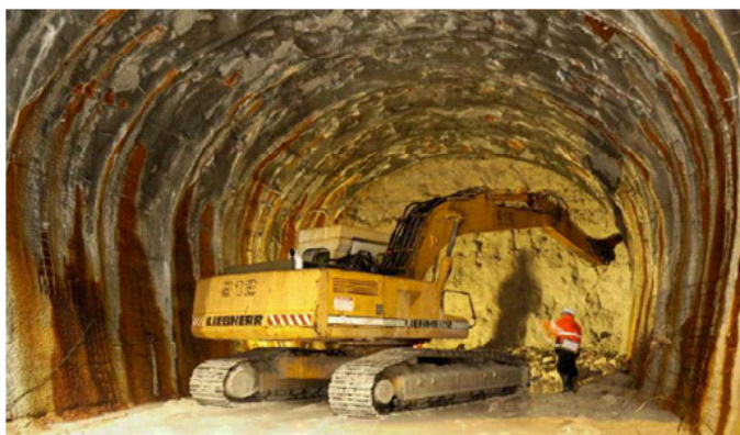
Construction of district heating tunnel under Copenhagen Harbor is the largest construction project in Copenhagen since the metro. The budget is 100 mill. Euro.
